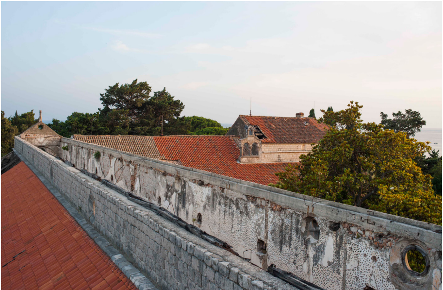
Figure 7. The roof missing from the central gallery of the Monastery and the damaged roof of the Abbot's (South) Wing.
