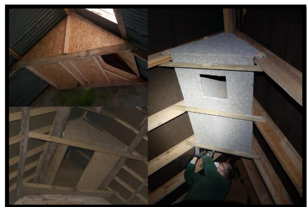
Figure 3. ‘Hot boxes’ of various design, installed into the apex of the roof interior at horseshoe bat roosts.
