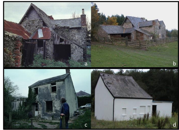
Figure 1. Examples of horseshoe bat roost buildings (Hendre cottage – a, b; Rose cottage front elevation (c) and rear elevation (d) when first discovered (a, c) and the same buildings following repairs and re-roofing (b, d).
