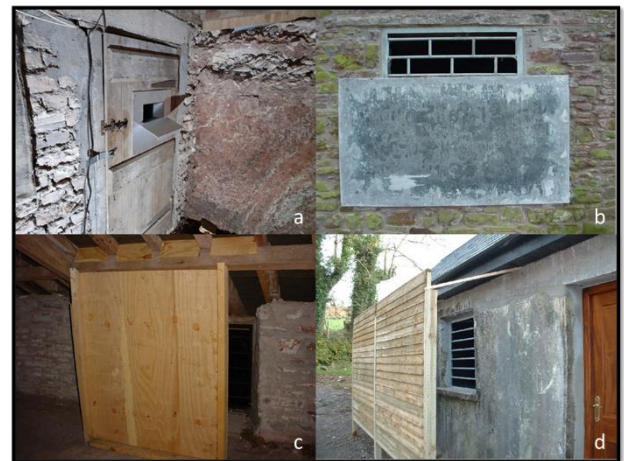
Figure 2. Entrance modifications to improve horseshoe bat roosts. Entrances can be made predator-proof by installing a ‘tip tray’ (a) and anti-climb surfaces (b). Grills can be installed to deter vandalism (b, d). Baffles can be installed to reduce draughts and light into the building (c, d).
