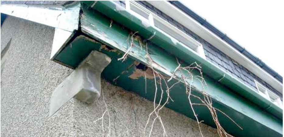
Photo: A potential access hole for a marten in a rotten soffit © Hugh Brown
