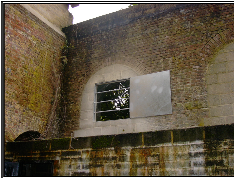
Figure 4. One of the two grilles in the eastern elevation wall – prior to re-roofing
