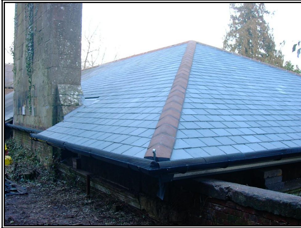
Figure 6. The final hip-end section on the southern elevation
